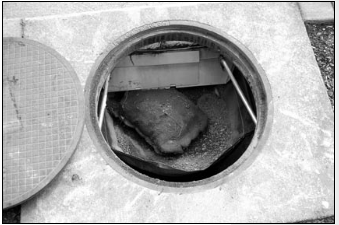
Top right: Special inserts made of Oregon wool are inserted into stormwater drains where they filter sediment and pollutants from the runoff.
